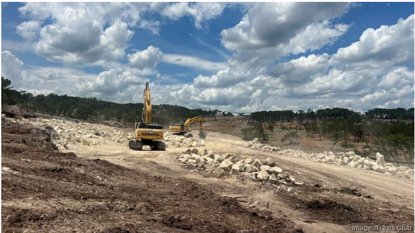
Infrastructure construction is underway at Travis Club.
